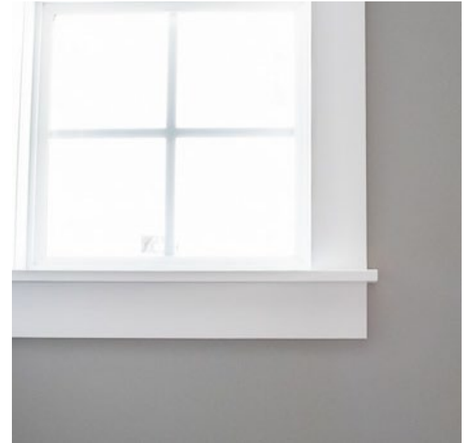
Window Sil Molding detail in main level bedrooms
